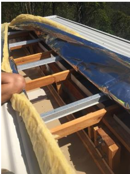
Figure 3 - Gable end blocks missing.
