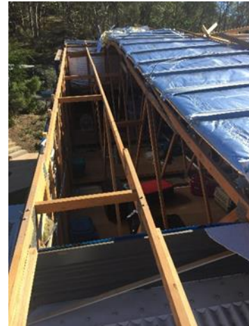
Figure 4 - Roofing upside down after a storm event.
