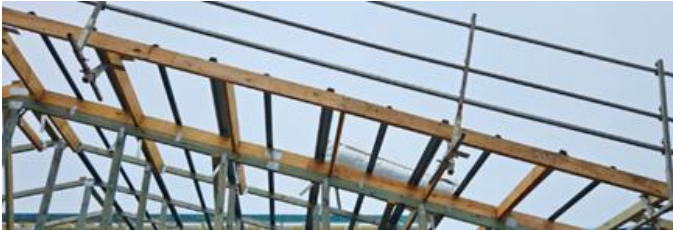
Figure 2 - Gable blocks plated to cut down trusses.
